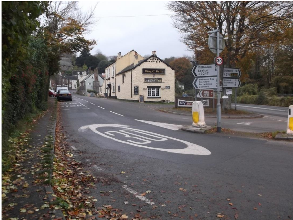
Photo 3.5 – 'Ring O Bells' Public House with car park and access
