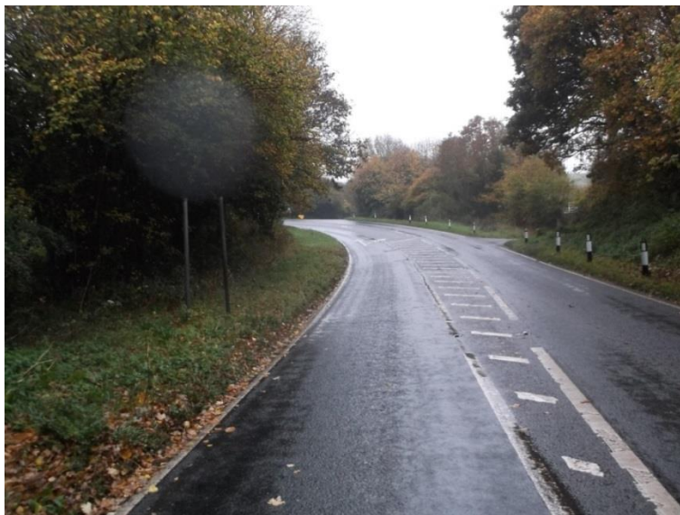
Photo 4.12 – Polscoe Bridge junction of A374 and B3247
