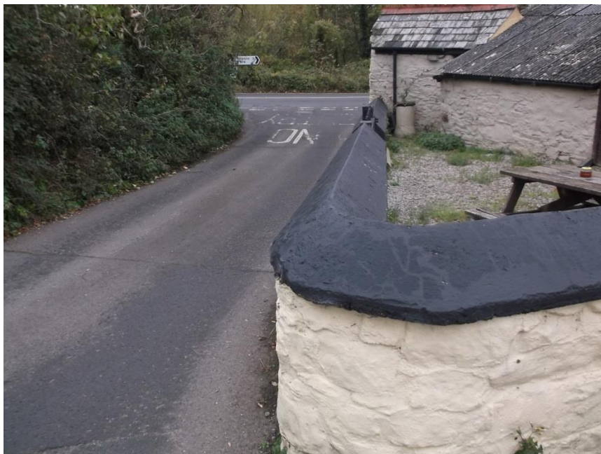
Photo 3.2 – Existing one – way link at Antony junction
