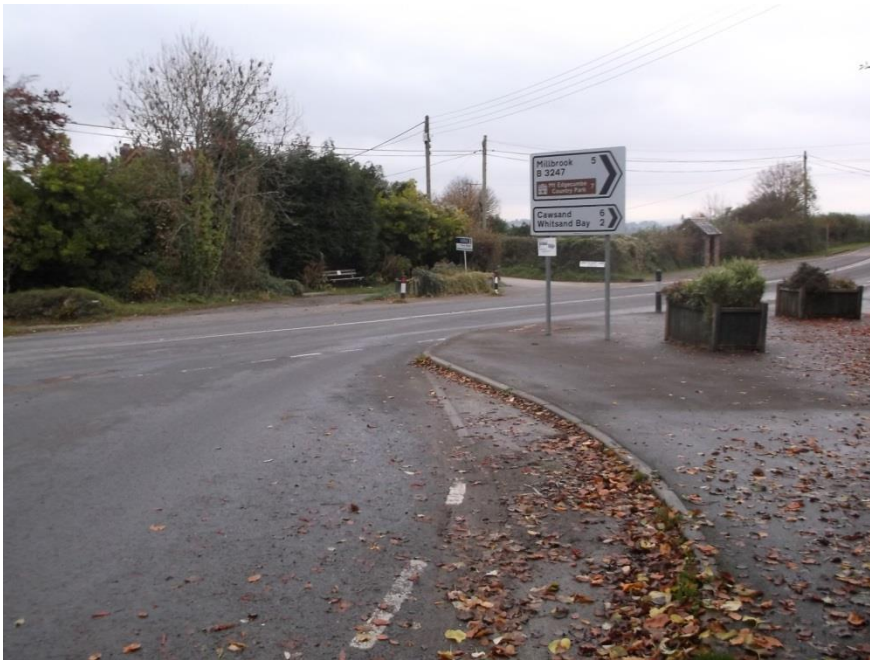
Photo 4.4 – Existing plate sign at right turn from the B3247 at Antony junction
