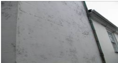
The render on the façade of this building has been lined-out to create the illusion of finely jointed stone ashlar
