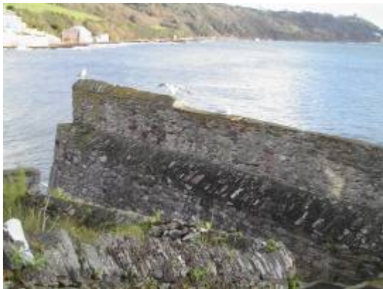
The thick sea wall above South Rock is constructed from slatestone
