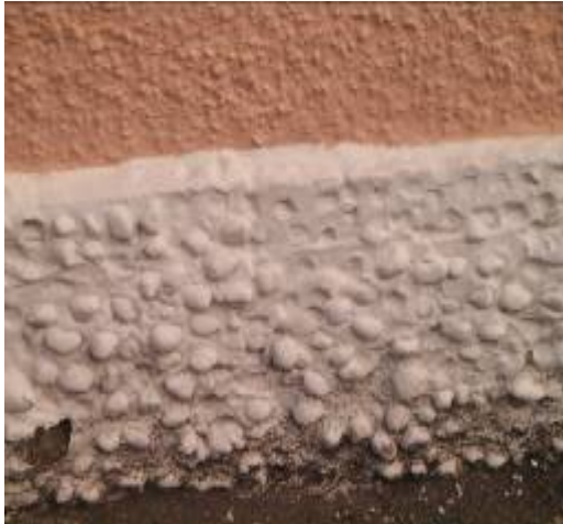
Cobblestones incorporated into the render are used to face a plinth
